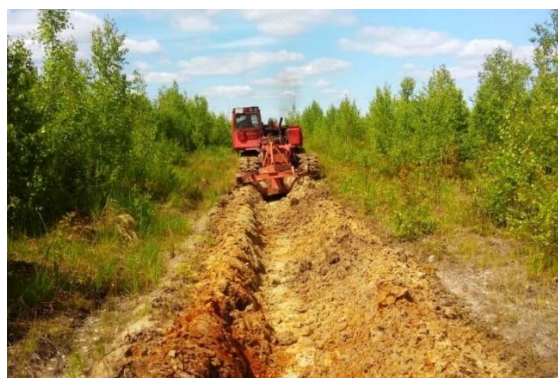
Figure 3. Creation of mineralized strip by mechanized method.
