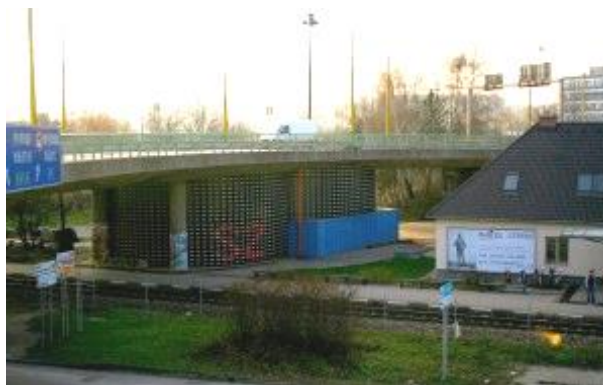
Fig. 8. S2 construction under roundabout in Žilina (Dobiaš, 2012).
